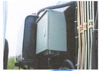
PLC Modular control box
